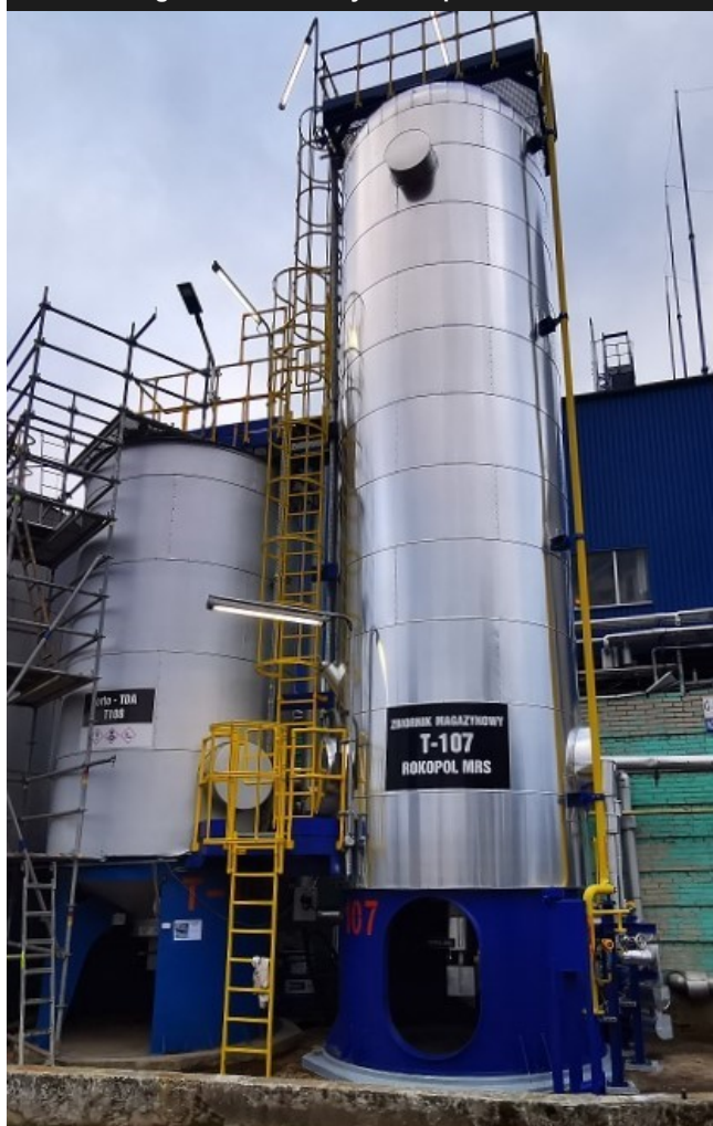
63 m 3 storage tank at the Polyol Complex
