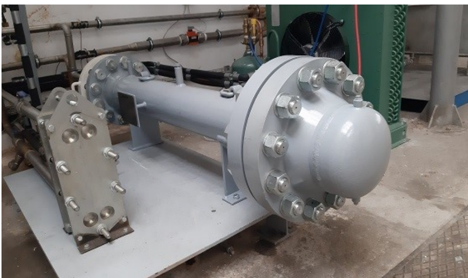
Gas cooler with titanium tube bundle
